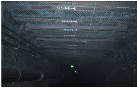
Fig. 73 Roadway support at the No. 5105 roadway
